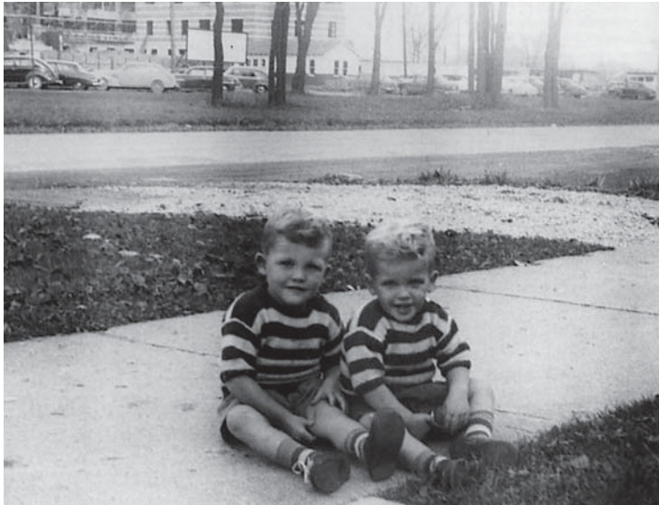
Richard and Mark, with St. John Hospital under construction in the background.
