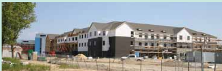
The short-stay hotel is also under construction.
