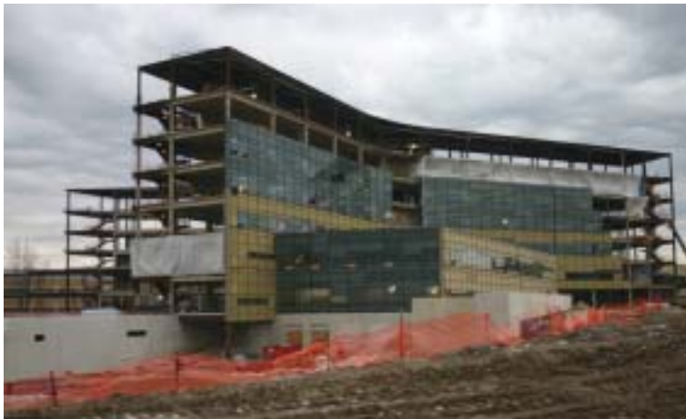
Construction continues on the new hospital.
