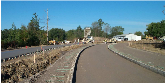
Concrete placement at the future new Main Entrance off Beck Road.
