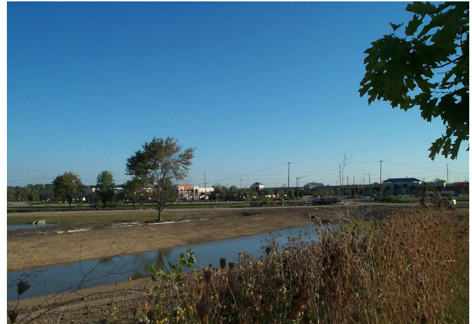
Looking north at the new storm water detention basin and section of the Ring Road.
