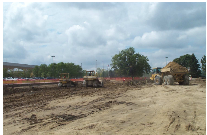
Rough grading of the new North Parking Lot.
